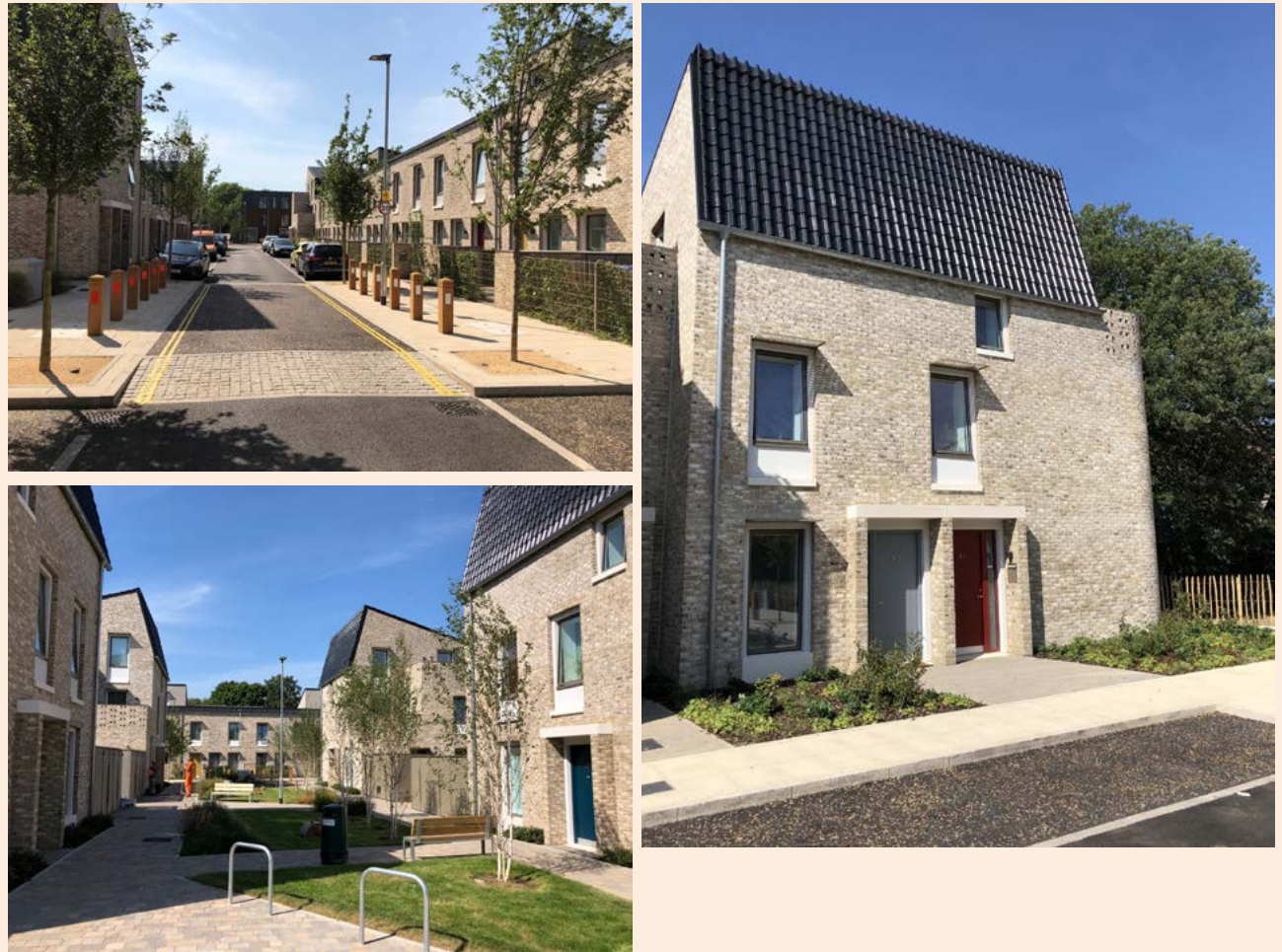
FIGURE 10: : GOLDSMITH STREET, NORWICH, DEVELOPMENT OF PASSIVHAUS HOMES (MIKHAIL RICHES ARCHITECTS)
